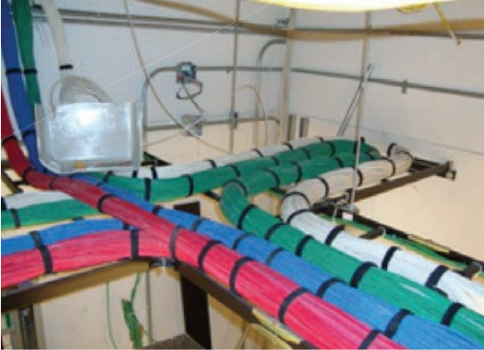
The intricate details of a cable path dressed in a Computer Closet are pictured above.
